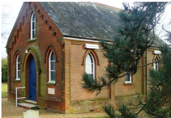
Picture 17. The Union Chapel, of early 20th century date apparently replaced a Primitive Methodist Chapel at Cheapside to the north.
